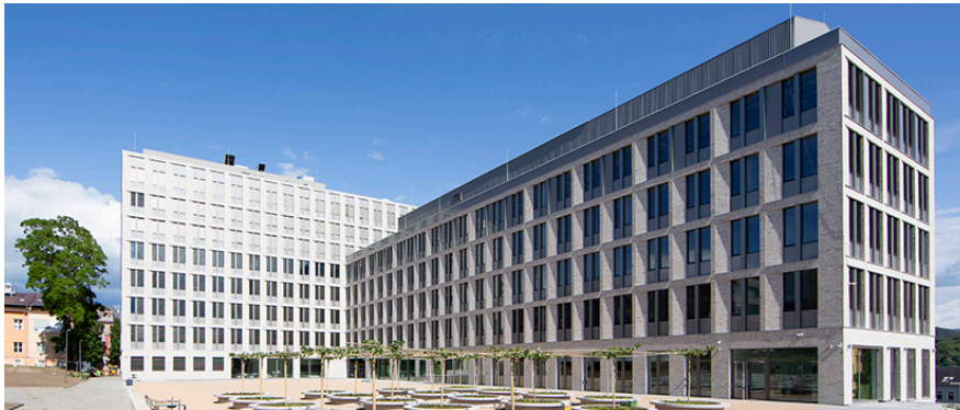
Main faculty building – Centre for Natural Sciences and Technologies
